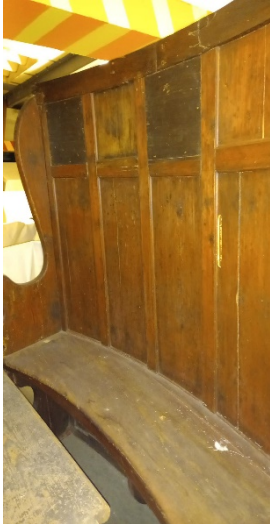
Settle back view of replaced panels
