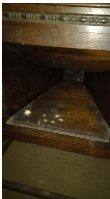
Interior of small cupboard with evidence of active furniture beetle.
